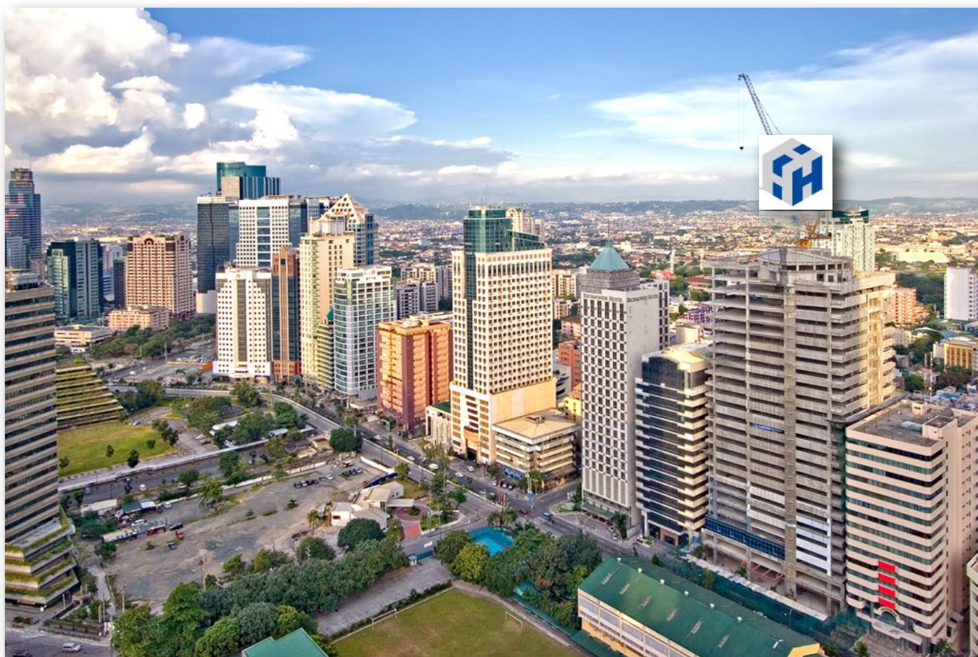
Frontage along San Miguel Ave.
